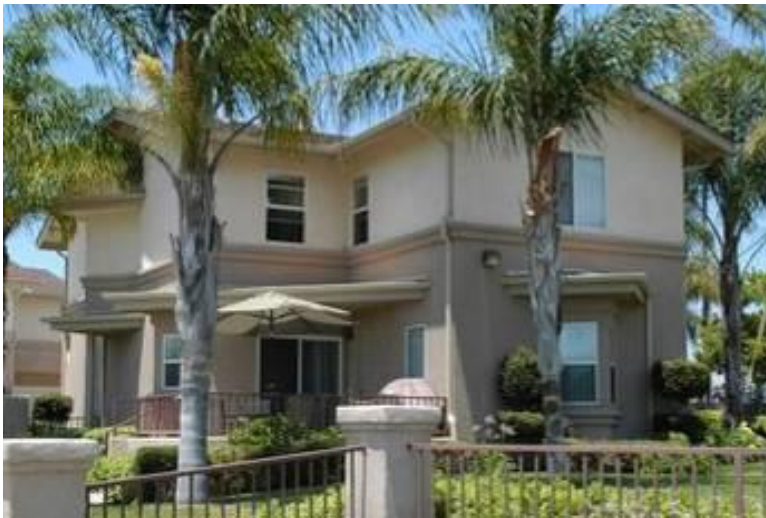
Orange considers development and rehabilitation of affordable family housing with emphasis on low and very-low income families as one of its highest priorities.
